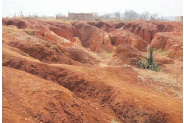
Figure 7.3 b : Soil erosion
