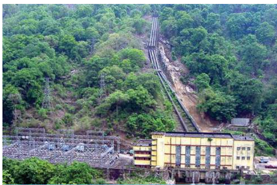
Hydro electric project - Pallivasal
