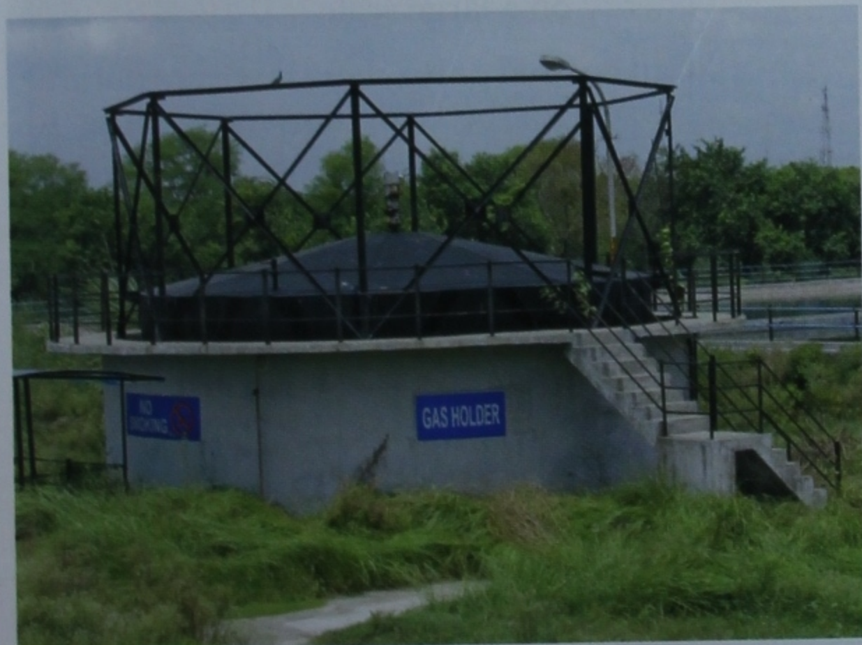
Fig. 5.16 Biogas holder in a sewage treatment plant
