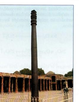
Fig. 6.6 The iron pillar at Delhi has not rusted for centuries.
